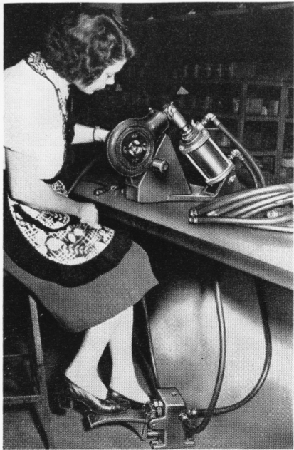
An operator (above) demonstrates how easy it is to work the foot pedal of Schrader's new Air-Operated Ferrule Contracting Machine. The use of air cylinder power
